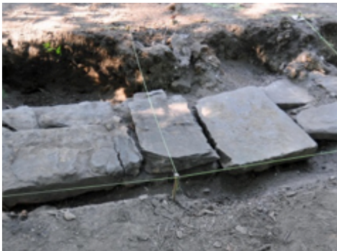
Foundation wall excavation
